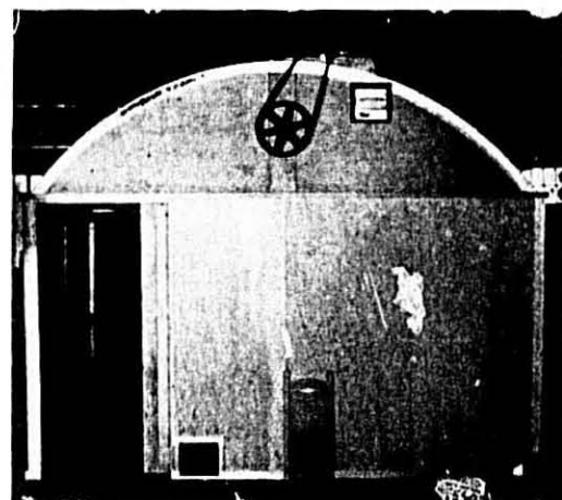
Exterior View—Lazzaro Drying Room
